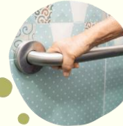
Grab bars in toilets for support
