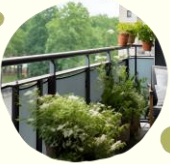
Additional handrails in balconies for support
