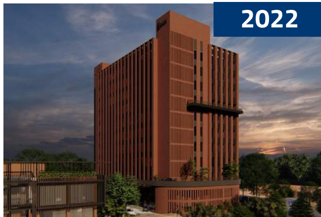
MAX HOUSE, OKHLA Phase 2 of campus expected to be delivered by 2023
