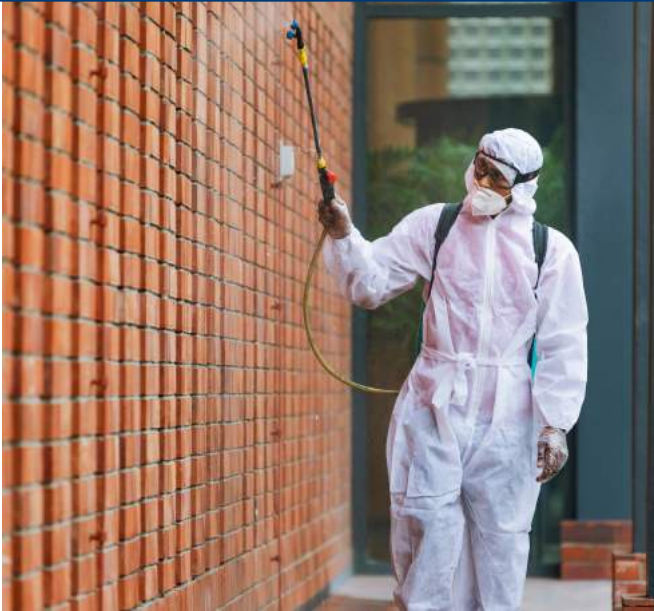
Deep sanitization of building premises using VIREX II-256
